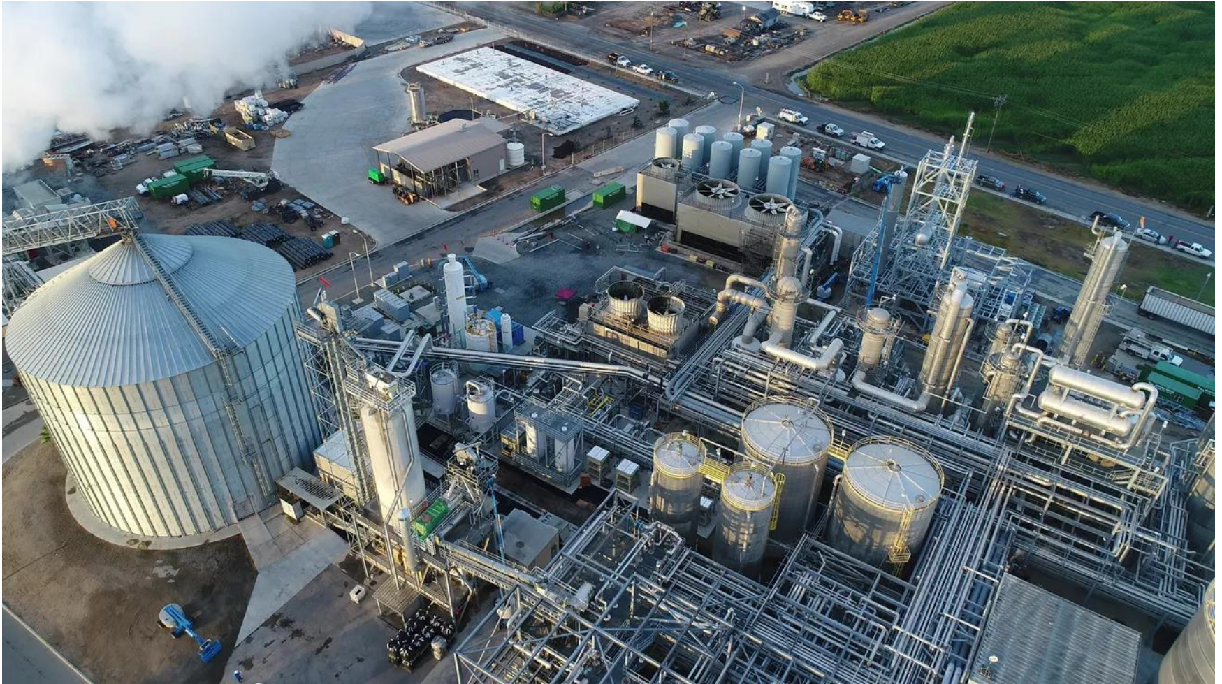
Calgren Dairy Fuels in Pixley, California, captures methane that would have vented into the atmosphere. SoCalGas
