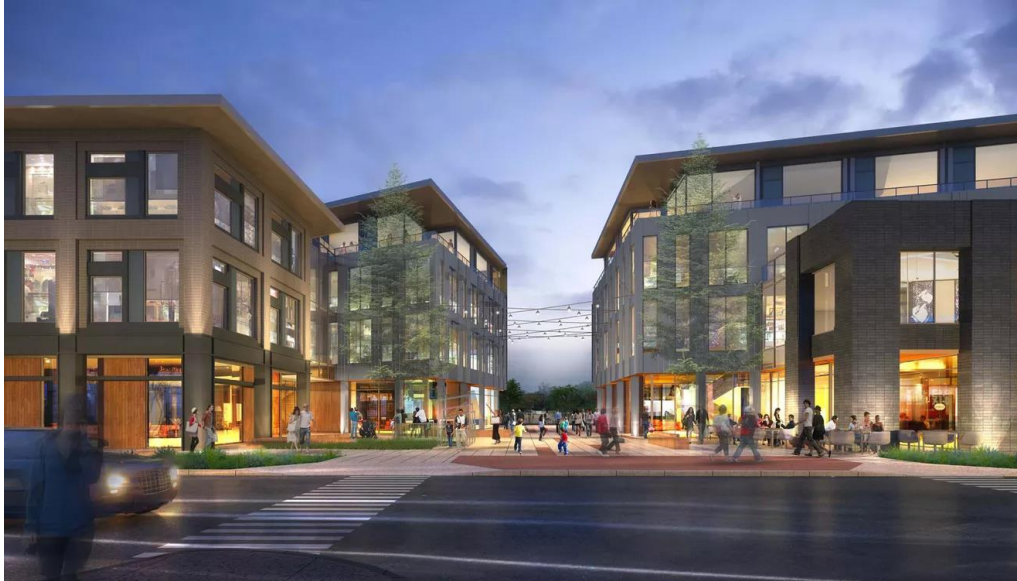
Boulder Commons, a new net-zero energy development in Boulder, Colorado, by Morgan Creek Ventures. RMI
